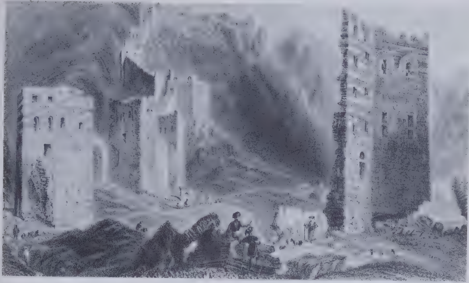
Antioch—The Walls, rebuilt by Justinian—6th century Engraving: Witt. Bartlett (London, 1837) (Photo: Dumbarton Oaks)
